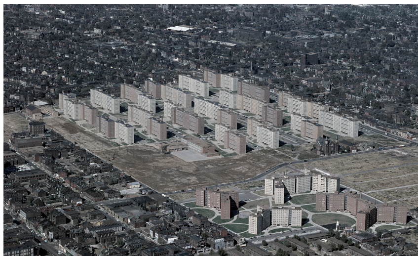
Pruitt Igoe: demolition on 15 June 1974 at 15:30. Source: Renato Saboya. http://www.flickr.com/photos/renatosaboya/7472167004
