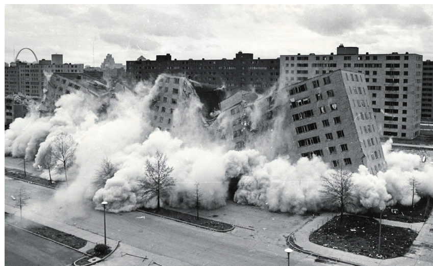
Pruitt Igoe: aerial view. Source: Renato Saboya. http://www.flickr.com/photos/renatosaboya/7472172108
