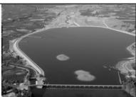
The anthropogenic effects of 'taming' the Aliakmon river are still further developing today as an additional dam upstream is planned for construction. The images above show the recent construction of an 'ecology focused' regulating dam (Agia Varvara dam) ensuring a steady flow regulated at 4 m<sup>3</sup>/s.
